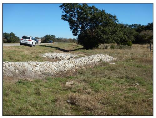
Photograph 26. Three visible best management practices at the Priscilla's Well KFA: roadway guardrails (left), rock gabions (center), and preserve fence (right).
