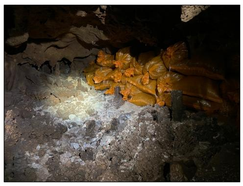
Photograph 44. Sandbags within Snowmelt Cave that were installed as part of cave stabilization efforts.
