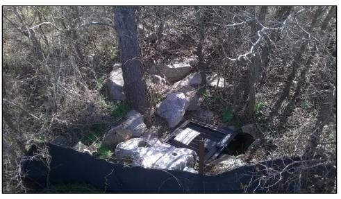
Photograph 8. Pemmican Cave silt fence filters stormwater entering the subsurface.
