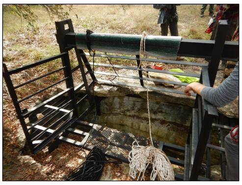
Photograph 9. Finalized steel A-frame being used to rappel into Coffin Cave.
